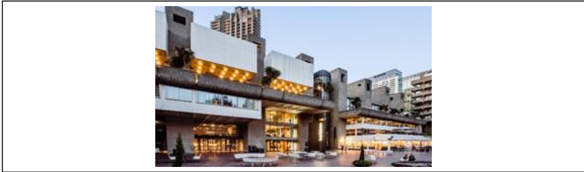
Image 2. Barbican Centre (Source: ArchDaily, 2022)
